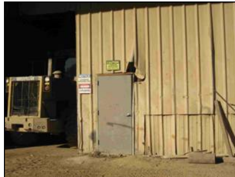
Note Heavy Equipment & Building Damage
